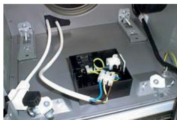
If the yellow/green wire is already present, fix it to the earth screw present in the hood. Connect the yellow/green wire in the remote suction unit to the suction unit earth wire in the same way.
